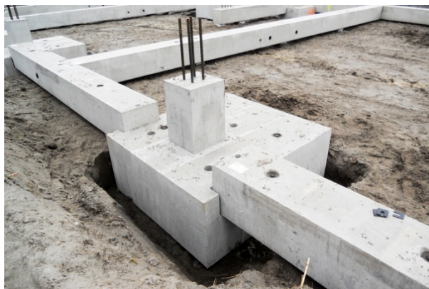
Figure 2c): Precast foundation with Tie beam slotted in place.
