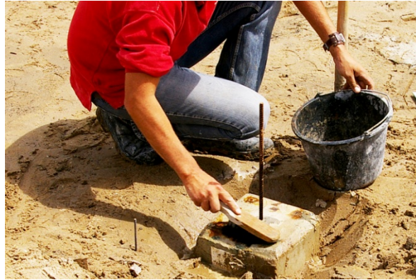
Figure 2d): Soil filled till top of the foundation pier.
