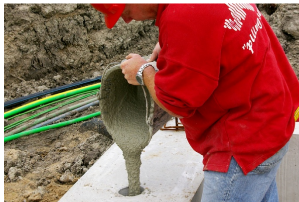
Figure 2f): Insitu grouting in the slots to make the system monolithic.
