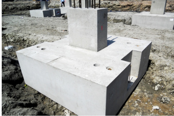
Figure 2a): Precast Foundation block.
