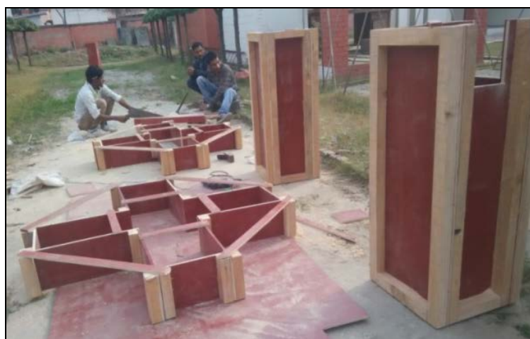
Figure 9: Formwork preparations on site at Rural Park CBRI, Roorkee.
