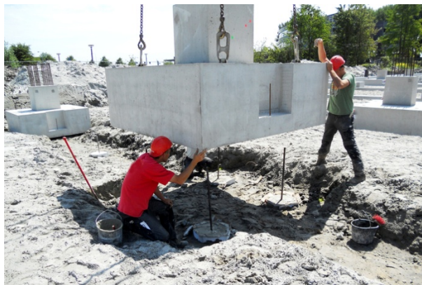
Figure 2b): Foundation block placed in the trench.
