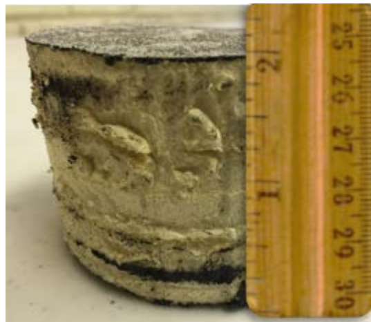
Figure 8: Core Sample #1 (Failing Core Sample)
