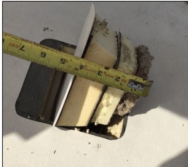
Figure 5: Roof "A" North Side
