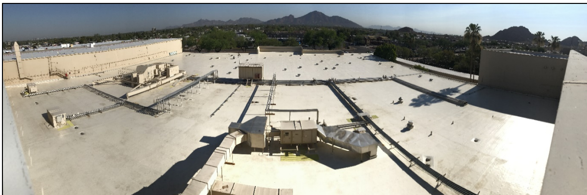
Figure 10: Roof “A” After
